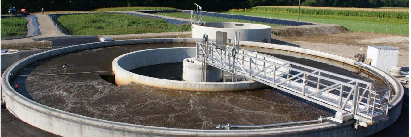
Figure 27: Aeration/anaeration tank and RBs behind in Dellach am Drautal<sup>29</sup>
