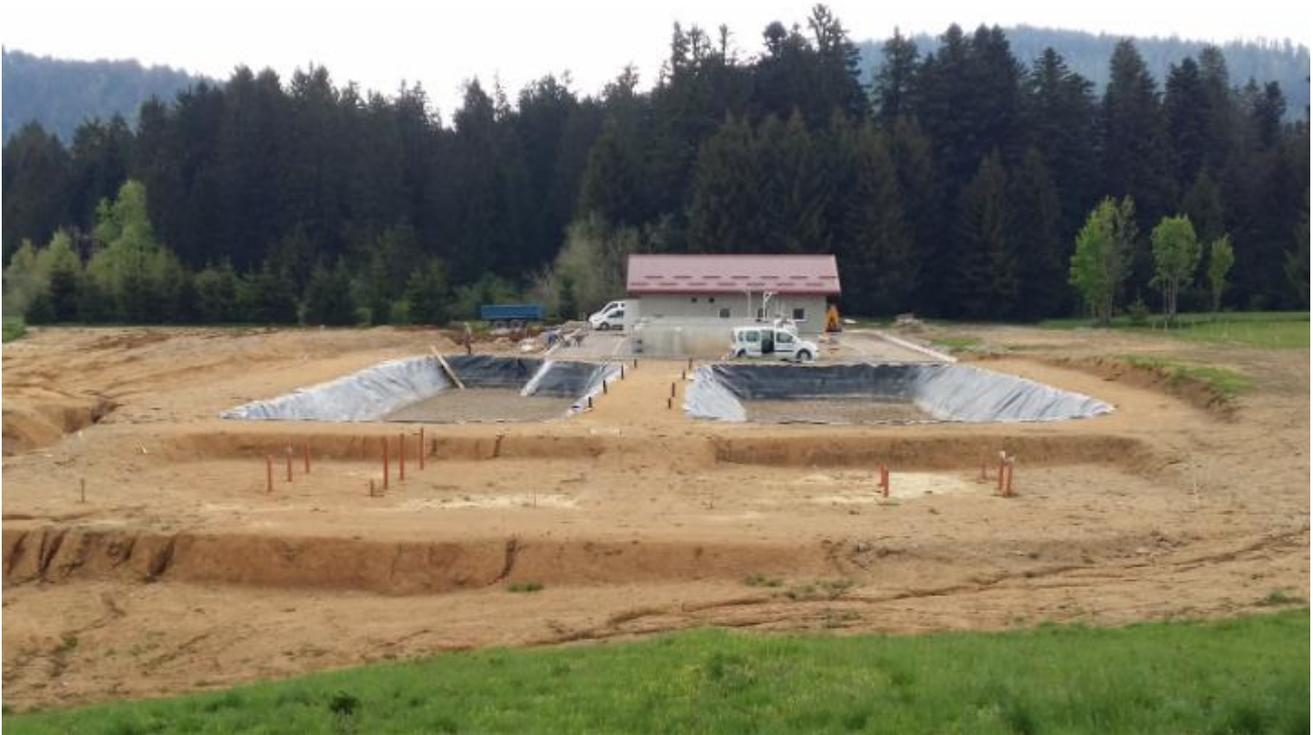
Figure 36: Two reed beds in Mrkopalj, after construction in 2017<sup>32</sup>
