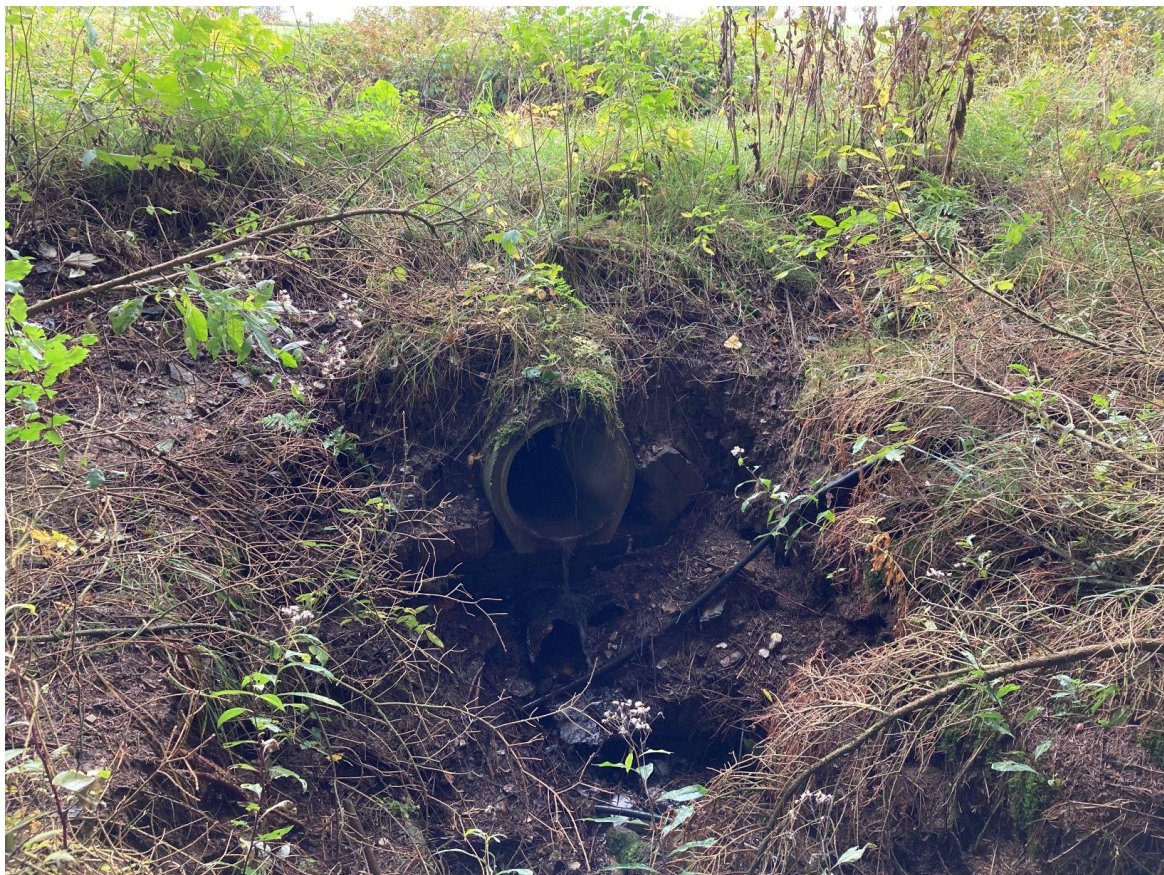
Figure 2 - Picture of one of the types of drainage ditches that currently runs through the study area. The drainage pipe transports water rapidly downwards, towards the Kyll, preventing it from infiltrating into the soil (picture provided by Lena Vitzthum, 9 October, 2020).
