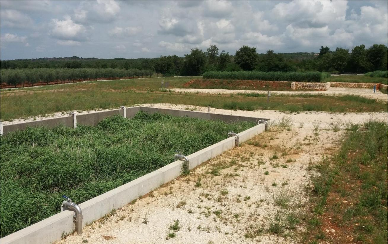
Figure 2: RB (front) with one of the five beds of constructed wetland (back) in Kastelir
