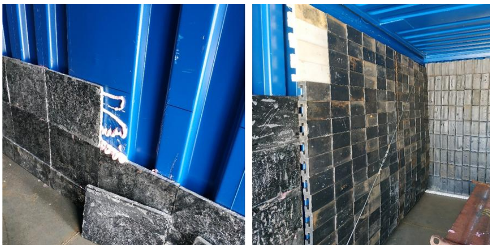
Figure 23. Neutron shielding inside of 20-foot ISO container
