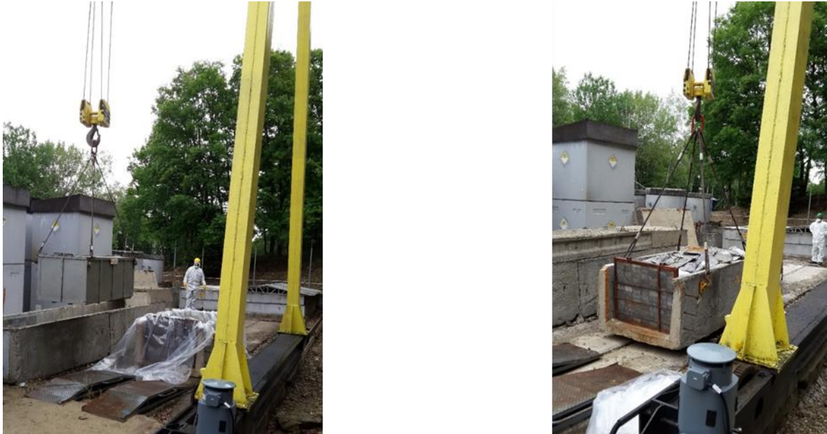
Figure 18. Positioning of the replica receptacle and positioning of crane
