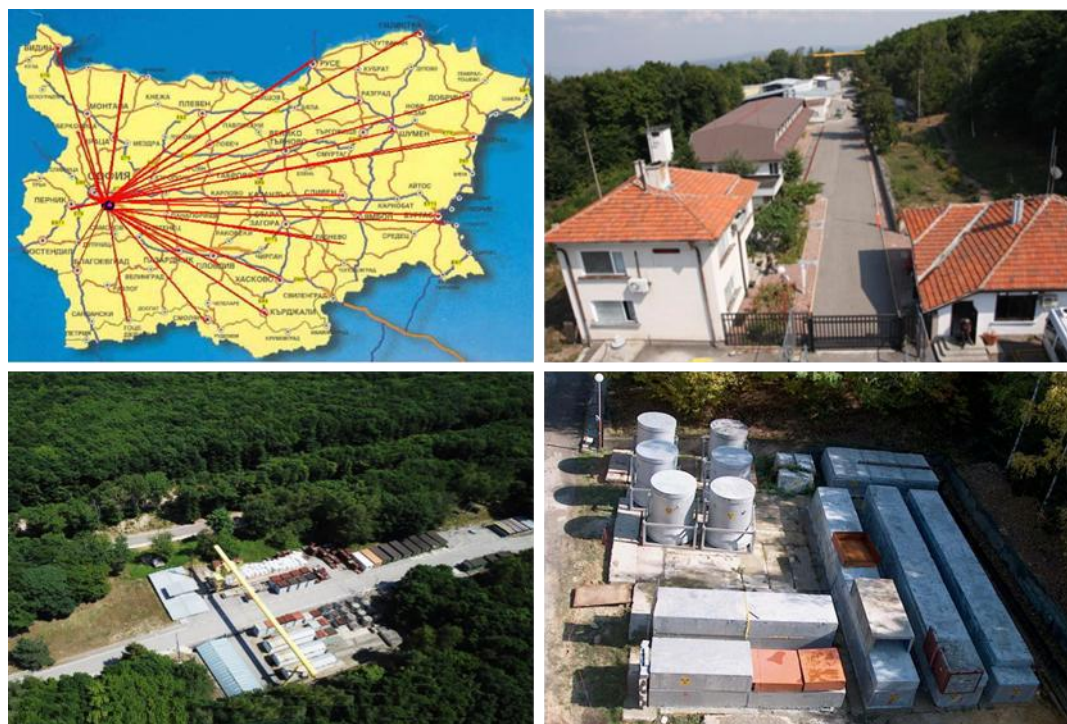
Figure 1. Location of SERAW's facility in Bulgaria: aerial views of entrance, site and storage area
