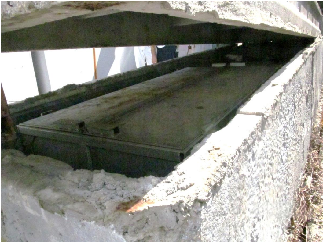
Figure 17. The Cs containing bale in place in its engineered solution
