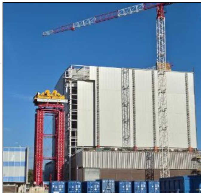
Adaptation of the existing steel structure for the steam generators and installation of an overhead crane on the top of the structure
