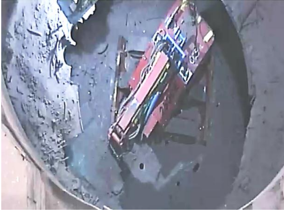
Excavator in reactor shaft on top of the platform
