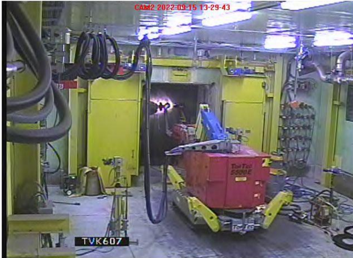
TOPTEC starts cutting the HLLW storage tank
