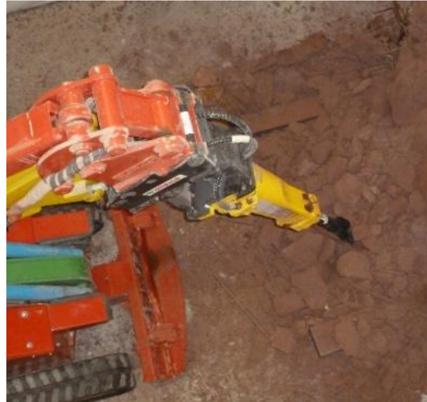
Hydraulic hammer attached to demolition vehicle
