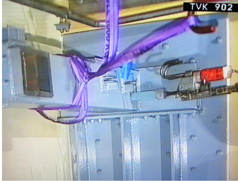
Hacksaw cutting reinforced steel structure
