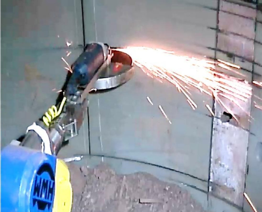
Cutting the formwork tank
