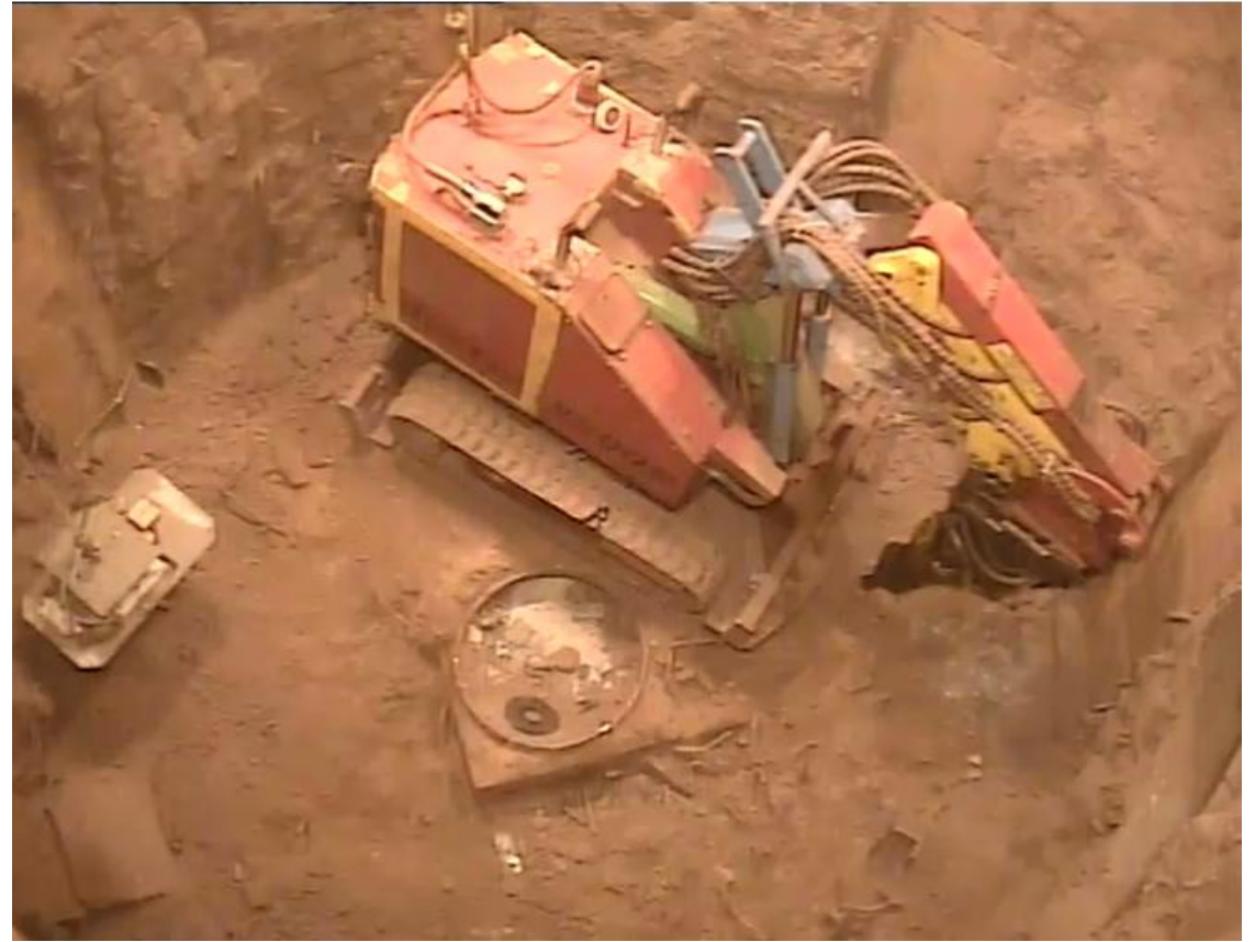
Excavator at bottom of the reactor shaft
