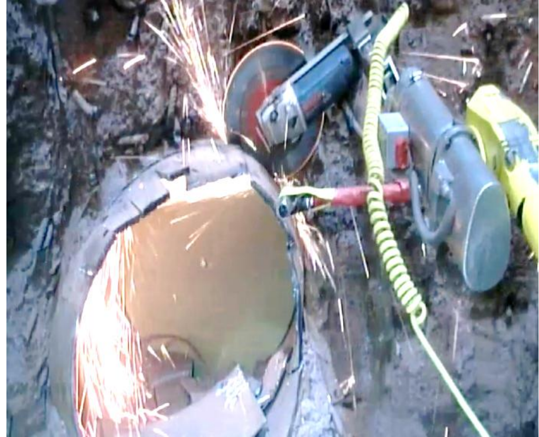
Cutting the outer edges of the sodium outlet pipes
