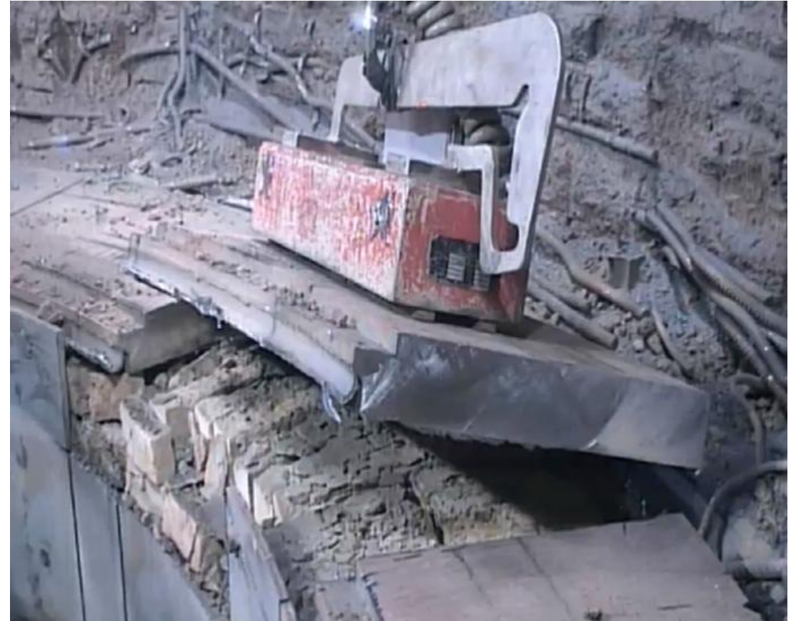
Picking up the first cut segment with a magnet
