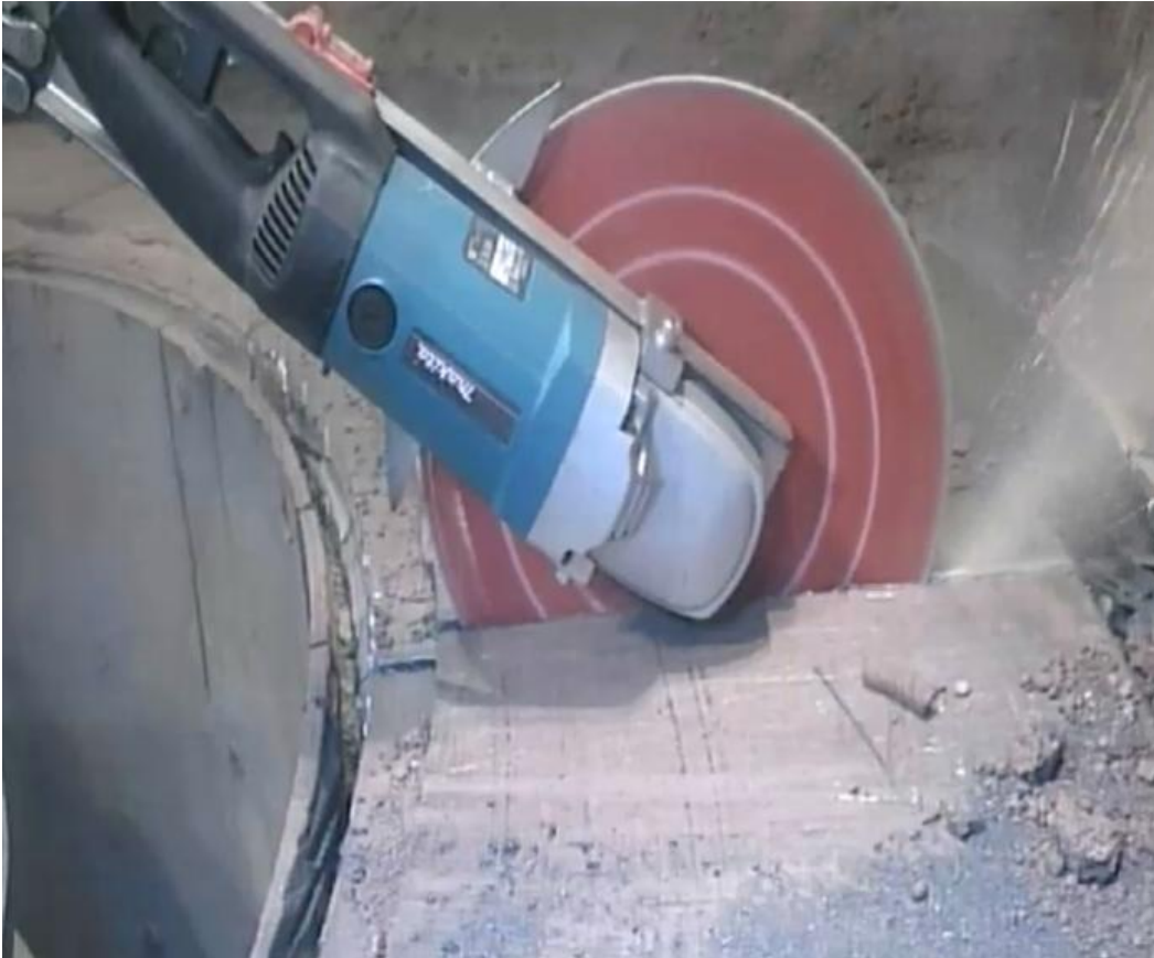
Remote cutting using an angle grinder(Cutting depth: 75 mm)
