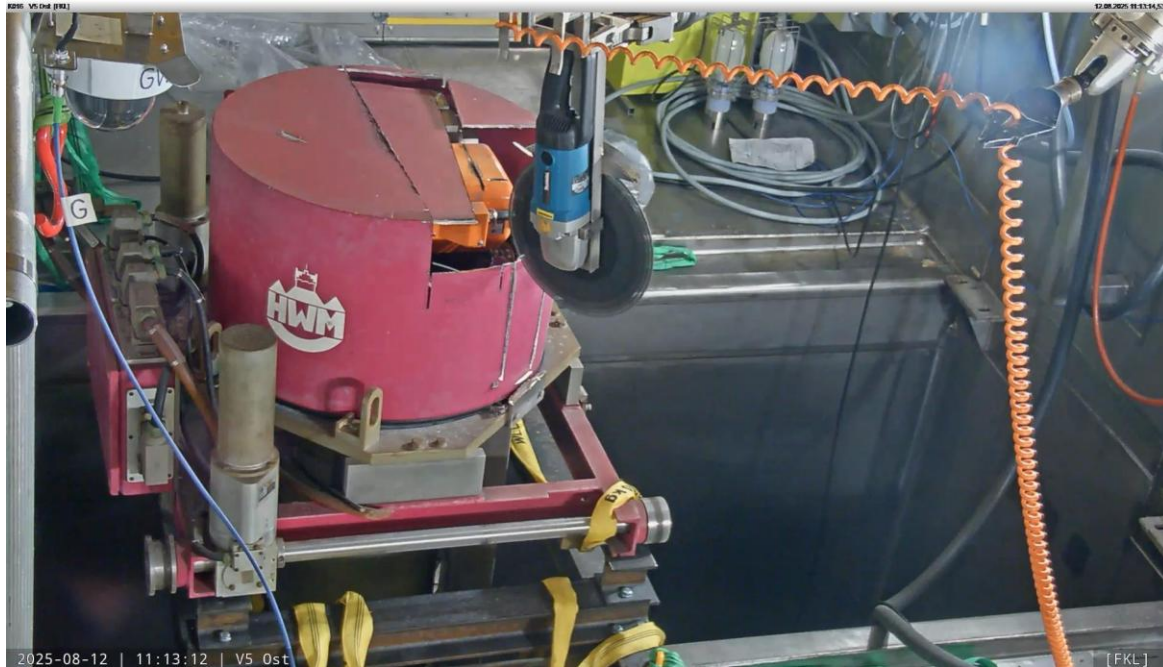
Cutting the manipulator housing
