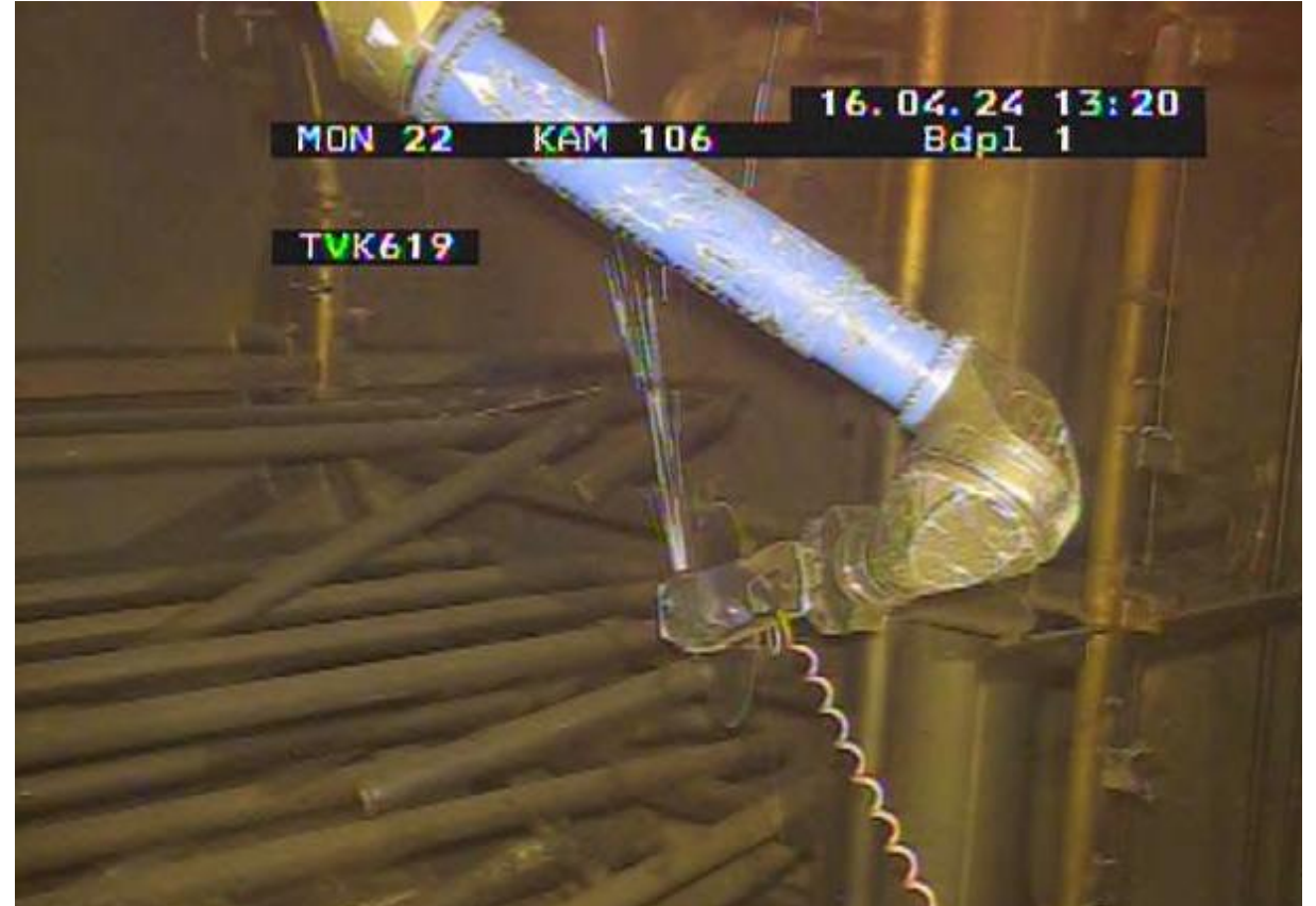
Angle grinder cutting couling pipes inside HLLW tank
