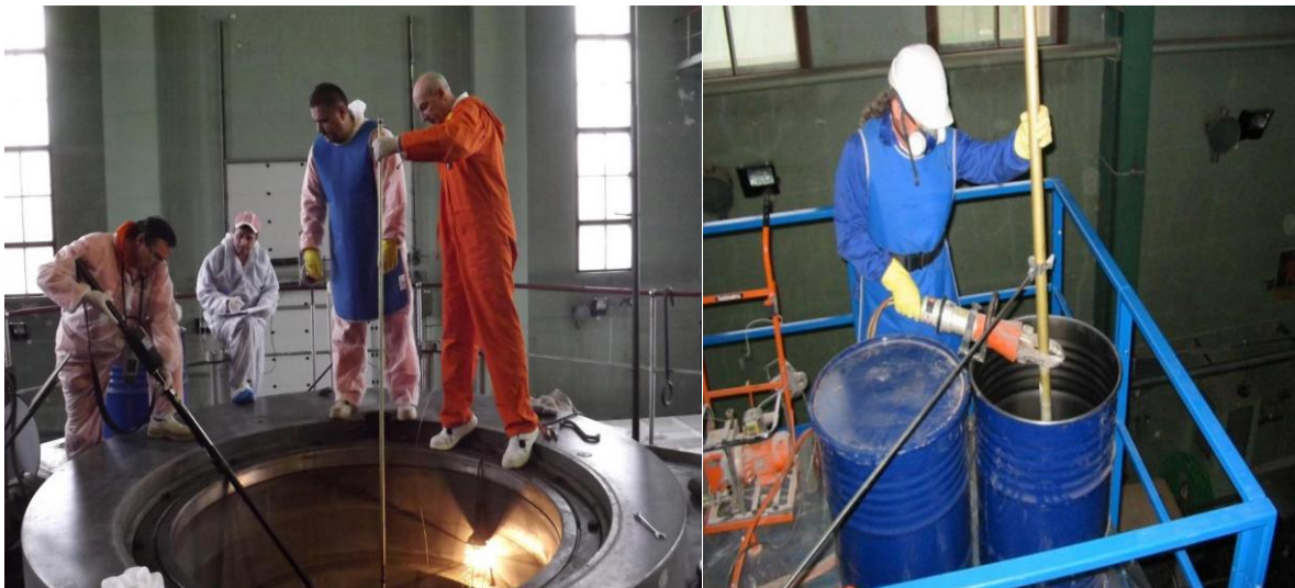
Figure 32: Lifting the control rod from the core (left) and cutting the control rods with the Holmatro scissors into 220 litre drums (right) [21]
