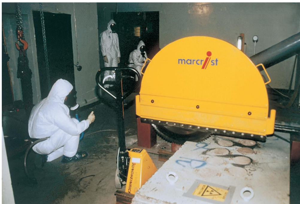
Figure 17: Creating new cell entrances using a diamond cable cutting machine (Top left); Concrete cutting using a diamond tipped blade saw (Top right); Dry cutting of cast iron shielding blocks using diamond tipped blade saw (Bottom) [1]
