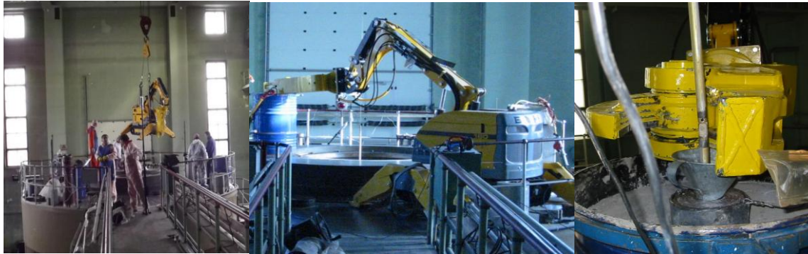
Figure 33: Placement and operation of the Brokk 160 [21]
