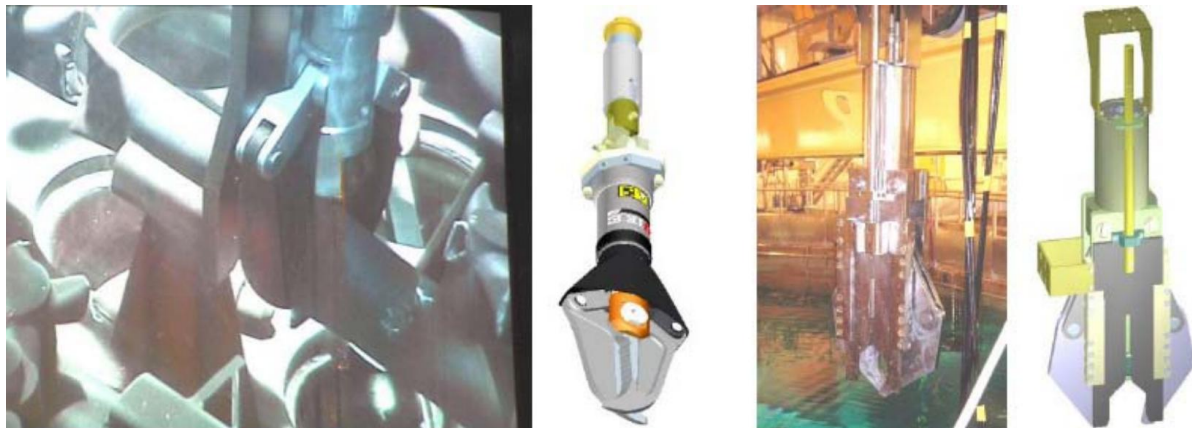
Figure 30: Shearing tools used to cut the core spray system and flat bars on the core grid [19]
