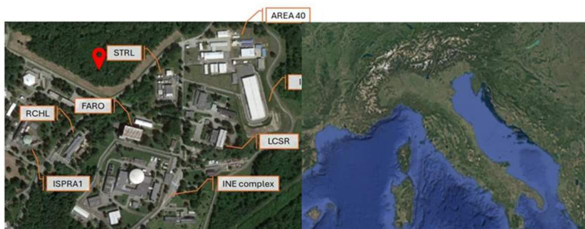
Figure 1. Aerial photo of JRC-Ispra nuclear installations
