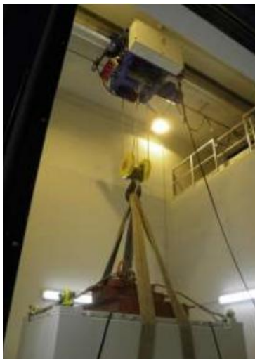
Figure 20. Crane used to lift CP-5.2 containers
