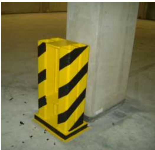
Figure 22. Column anticollision beam
