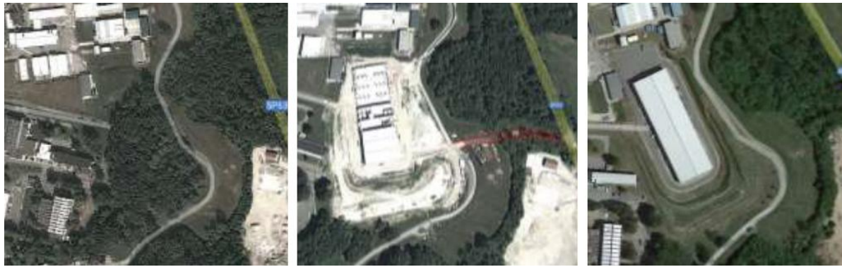
Figure 9. Timelapse of construction at Area 40 (left to right: before - temporary entrance in red - after)
