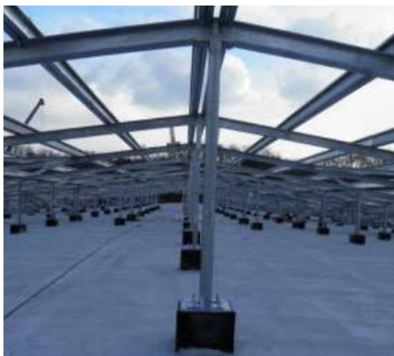
Figure 16. The first metallic roof during construction
