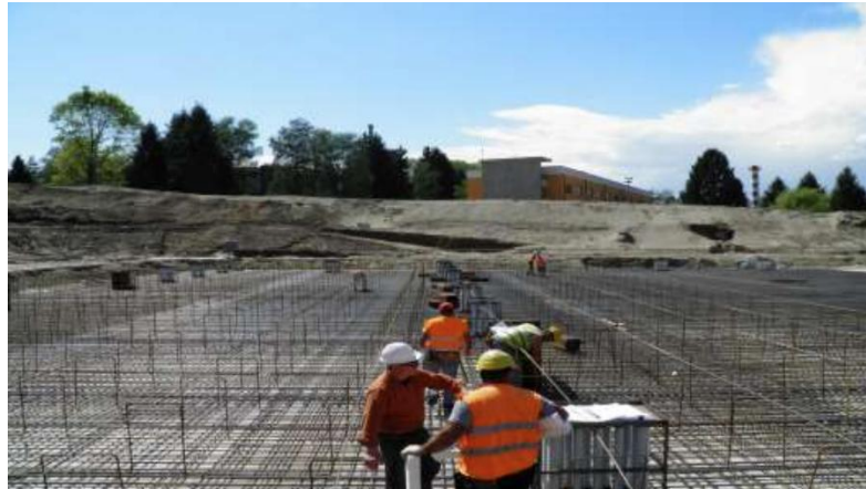
Figure 12. View of the foundation's steel reinforcement
