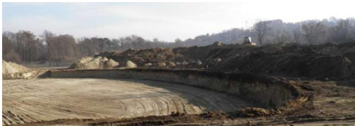
Figure 10. View of removed foundation soil
