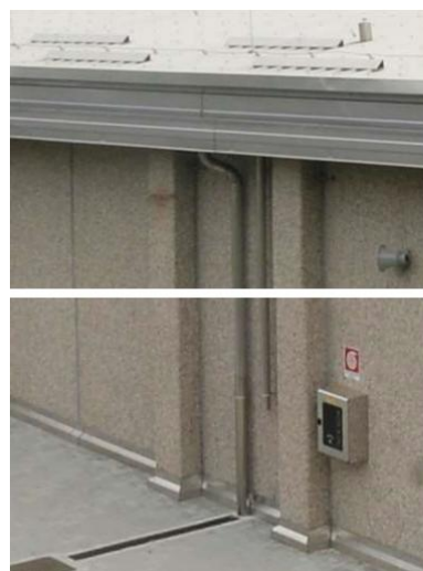
Figure 17. Details of rain drainage
