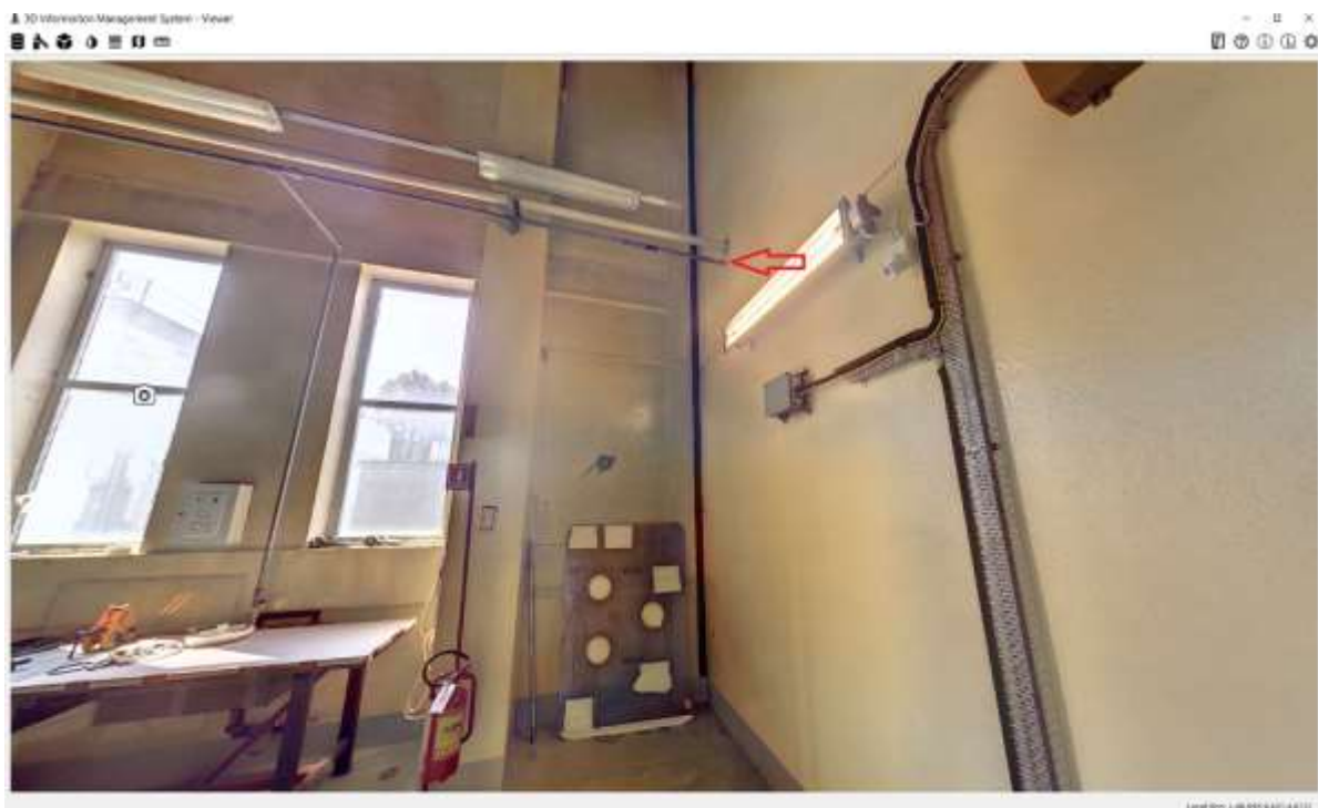
Figure 28: Continuation of the same pipe in room 4413 of ADECO, here the system is identifiable by colour coding the penetration is again marked with a red arrow
