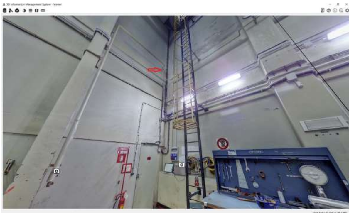
Figure 27: A pipe without system colour coding in room 4301 of ADECO pool viewed in 3DIMS continuing into another room through penetration marked with a red arrow
