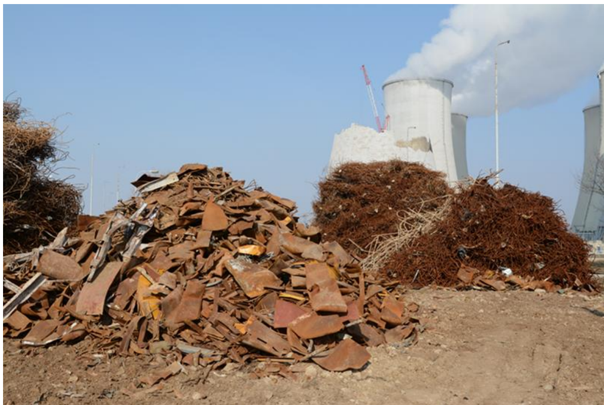
Figure 6: Metals separated from the reinforced concrete
