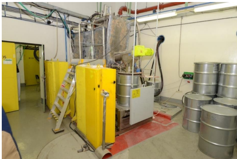
Figure 12. Drainage equipment shielding
