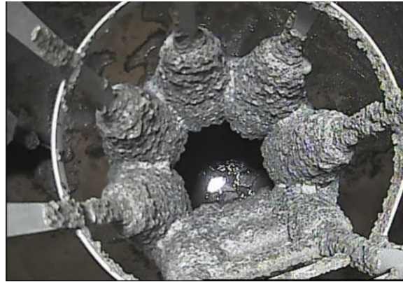
Figure 3. Radioactive concentrates in the storage tank
