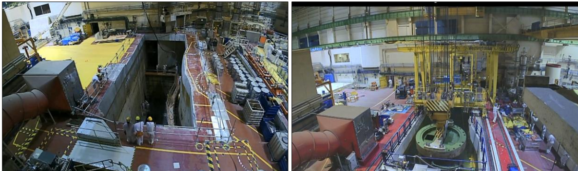
Figure 2. Construction of the wet-cutting workshop (left). RPV in the wet-cutting workshop (right)
