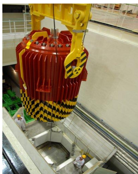
Figure 30. C-30 Container used to transport the shielding assemblies
