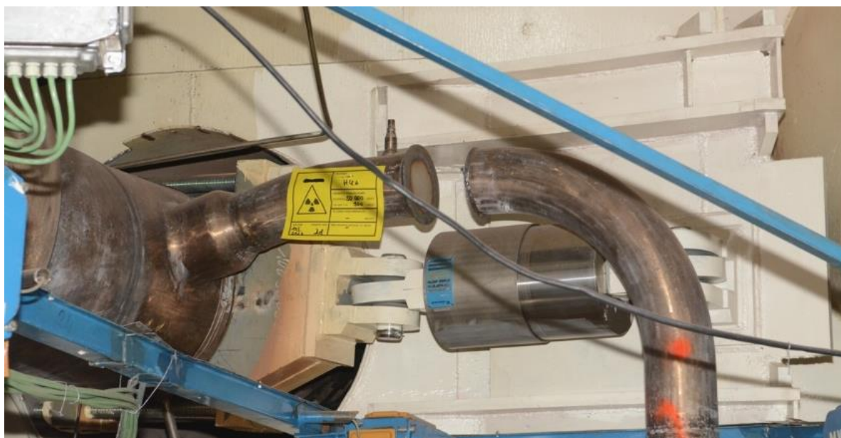
Figure 10: Modification of the blind pipe of the low-pressure emergency filling of the primary circuit.
