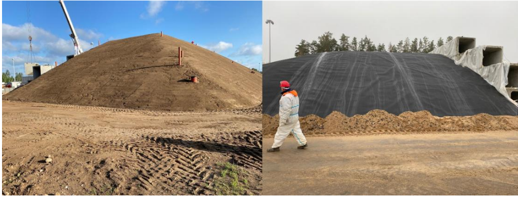
Figure 5. The foundation at different stages of development
