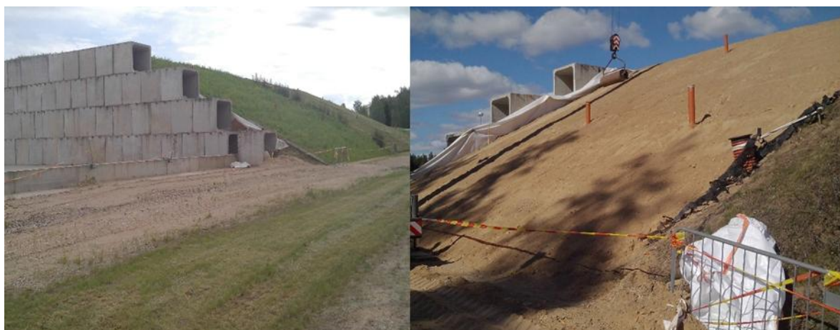
Figure 3. Snapshot of works in progress
