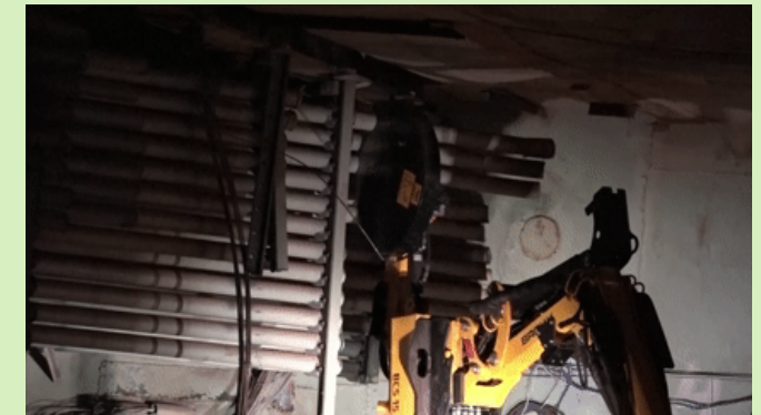
Cutting pressure pipes
