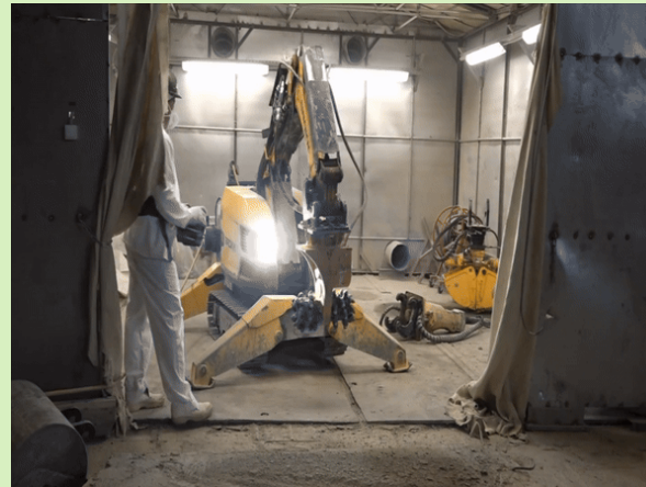
Hydraulic breaker replacement
