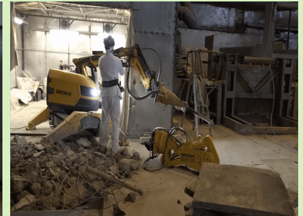
Metal shear replacement
