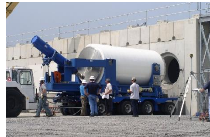
Figure 9. Process of introducing a cask into the HSM [4]
